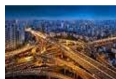
High Mast Lighting
